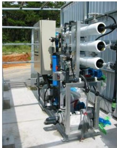
5)  $40 \text{ m}^3/\text{day}$  RO unit for seawater desalination
